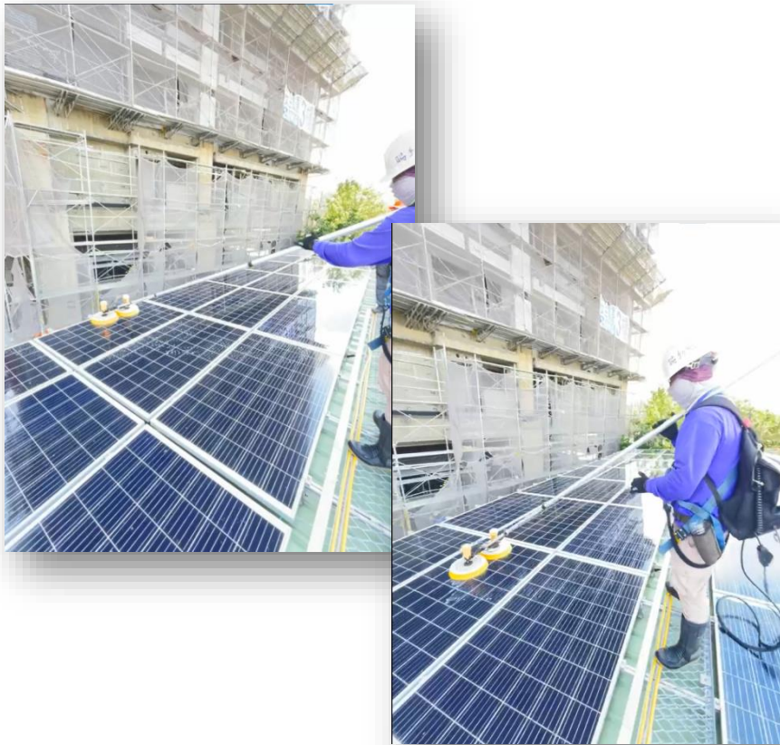
Cleaning PV module
