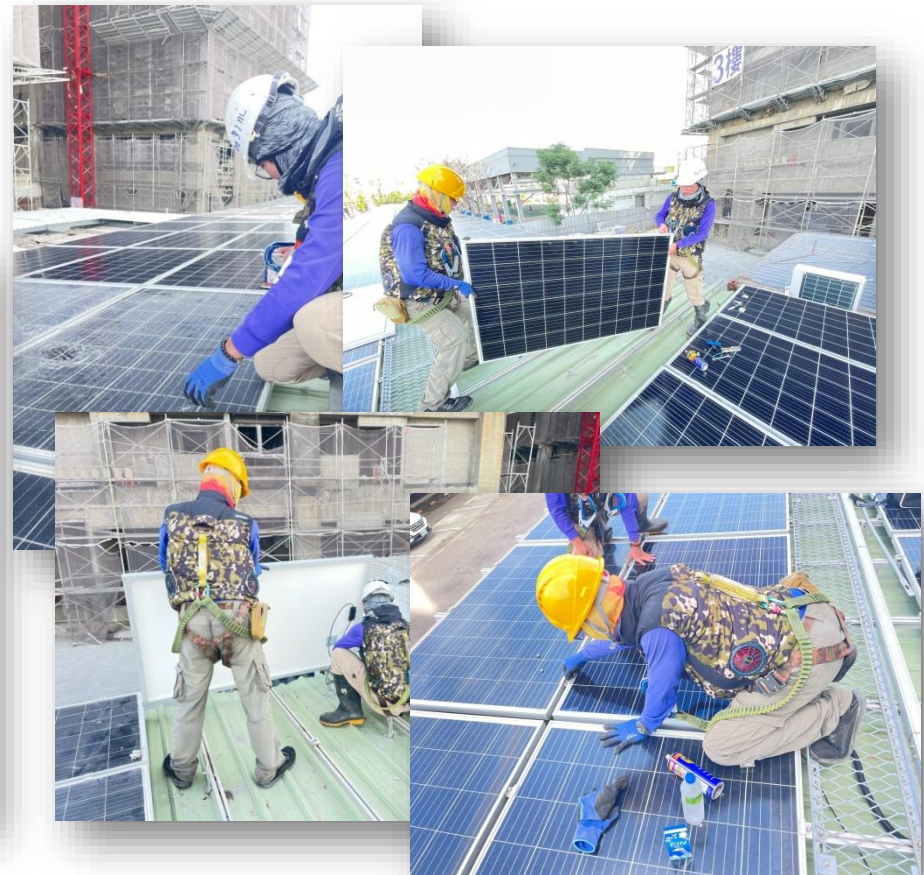
Replacing PV module
