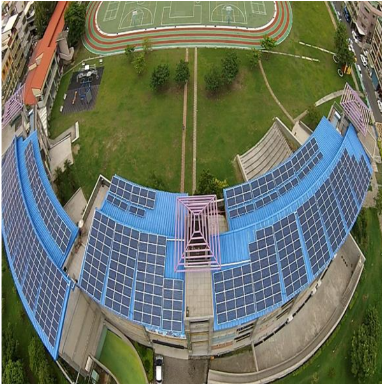
Wun-Shan Elementary School, Kaohsiung
